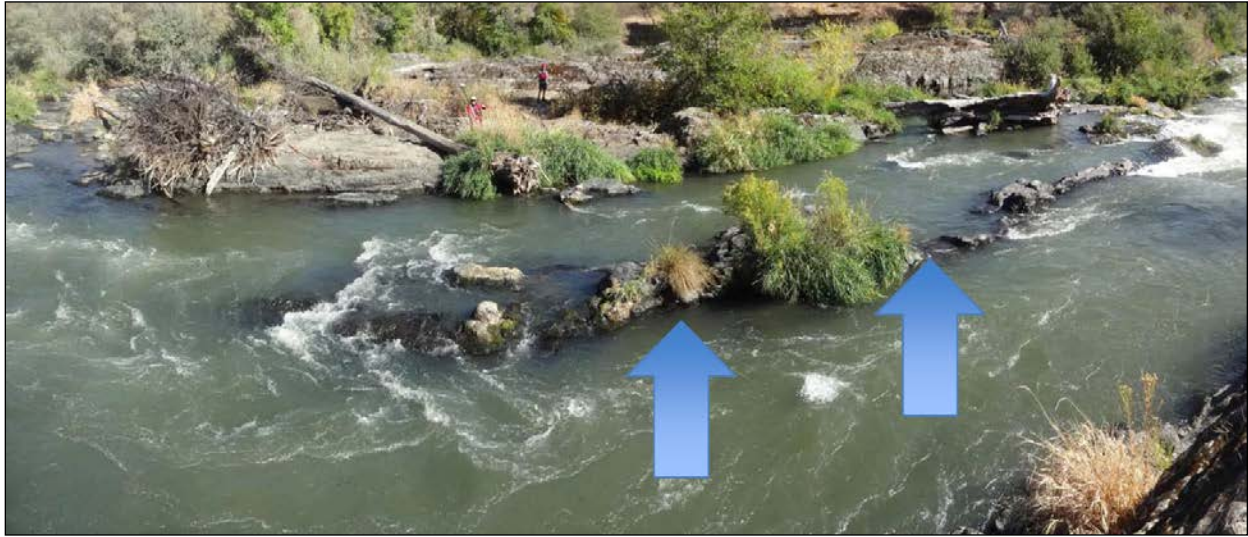
Figure 6. Selective rock removal to improve navigation and safety (Gill Hill project site).
